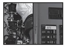
Use the transfer handle to move the main contacts in the transfer switch to the UP (utility) position. Switch the 2-pole breaker ON in the distribution panel.
